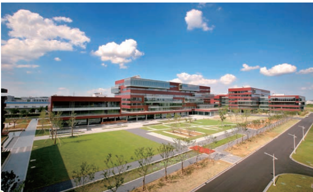
Production base of NJCTT
