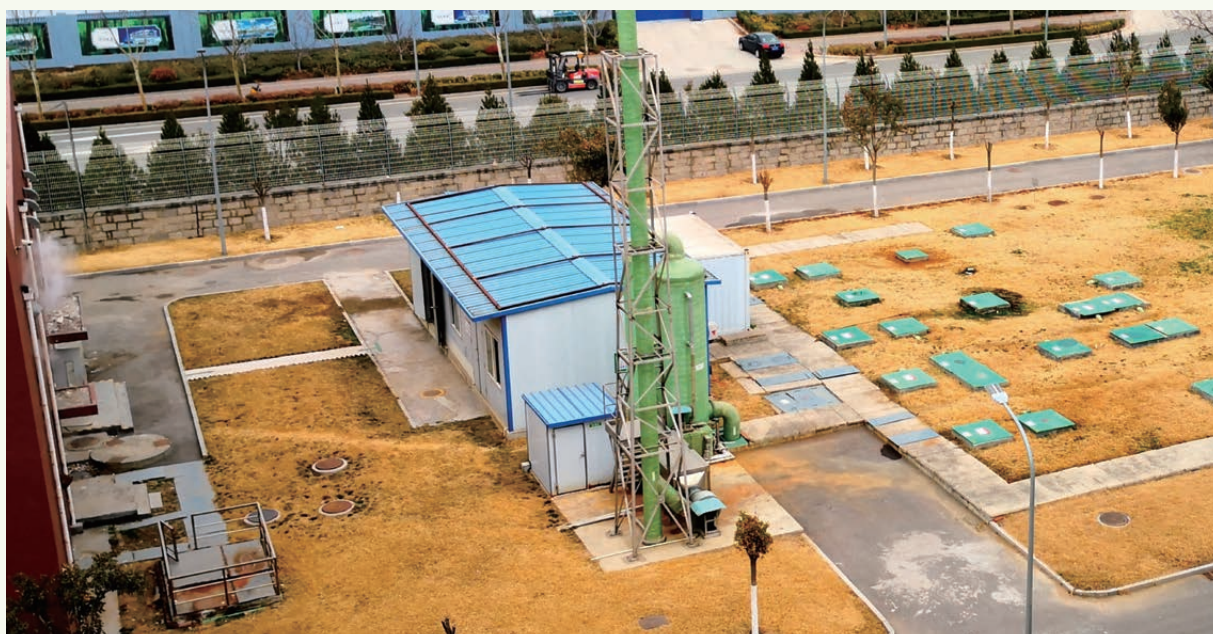
The wastewater treatment facilities of CP Pharmaceutical (Qingdao)
