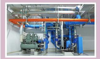
The 7-12°C refrigeration unit was turned off in winter when the weather was cold, and the valve was switched to the standby cooling tower system on the roof of Building No. 9. The heat generated by the 7-12°C system was absorbed by the standby cooling tower to reduce the energy use of the entire system. According to the compressor and pump power of the 7-12°C system and the winter switching time (3 months for one workshop), 180,000 kWh of electricity had been saved for the whole year.
